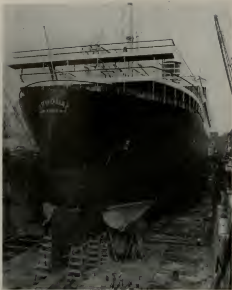
The 20,183 ton Moore-McCormack Line Uruguay, gets a final daub of paint around the rudder at the Brooklyn Division of Todd Shipyards Corporation.
